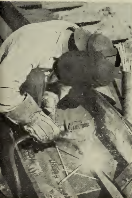
Steel Worker (SW)
